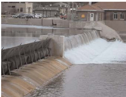
A view of the Waverly inflatable dam from the west.
