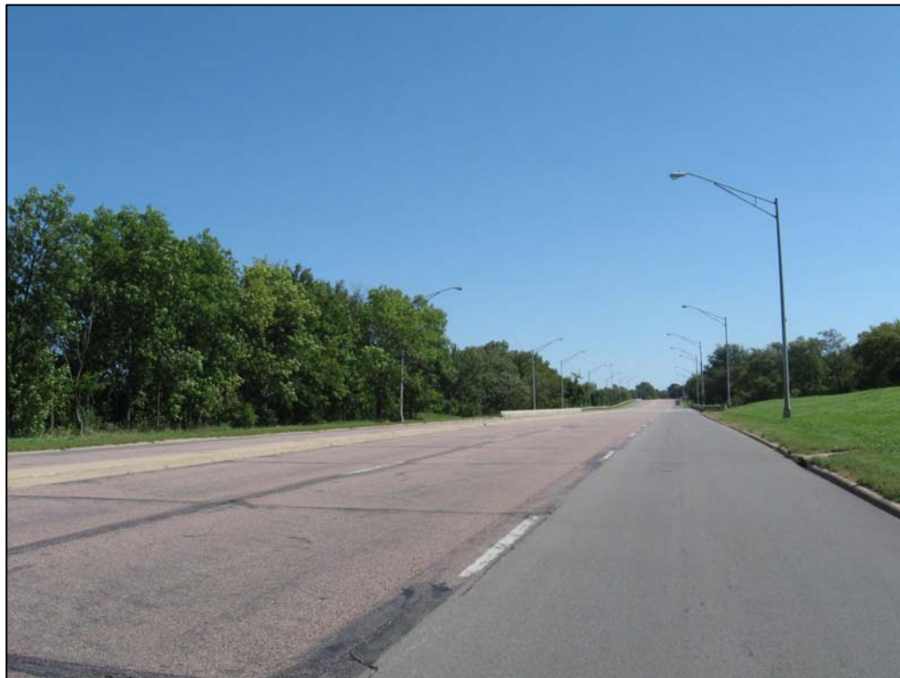
Looking east from Fletcher Avenue. Traffic volumes drop off considerably in this segment.
