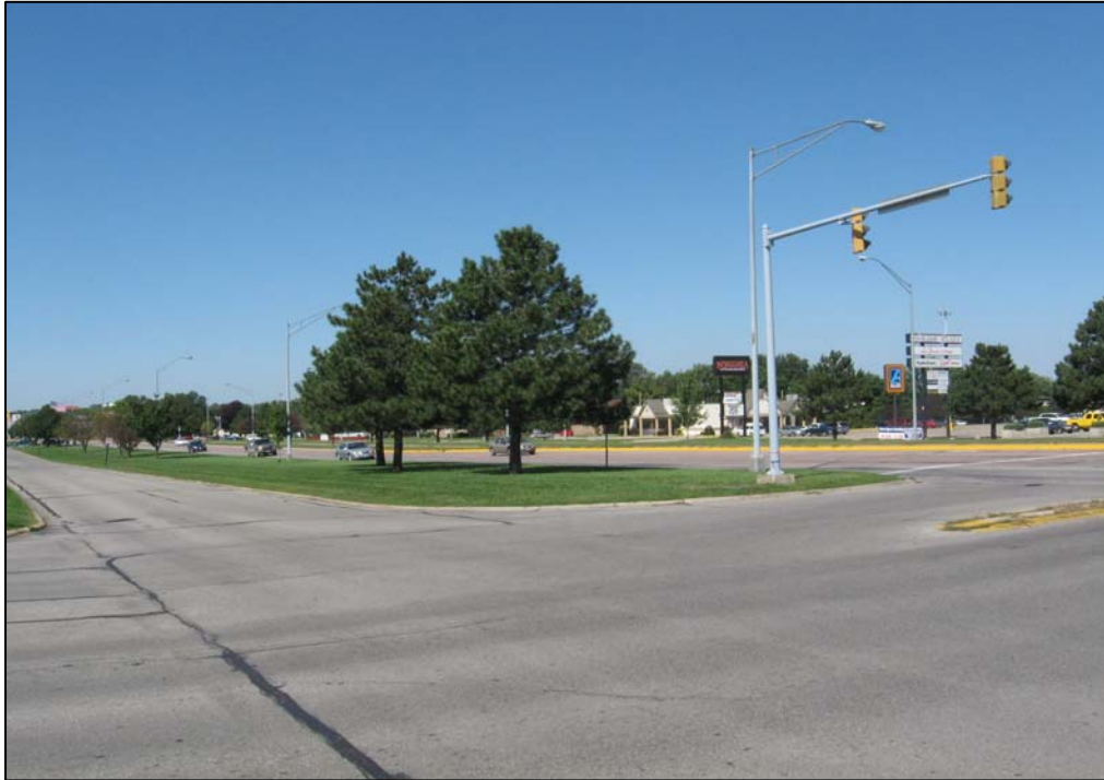
Typical view of frontage road and median near College Square Shopping Center.
